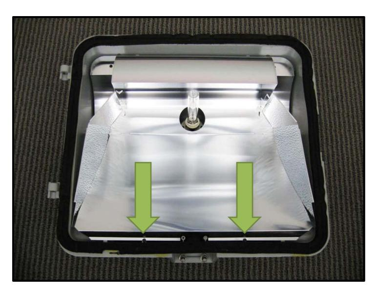
1. Disconnect electrical power before opening luminaire. Open Glass Door. Remove Reflector Screws and Main Reflector.
